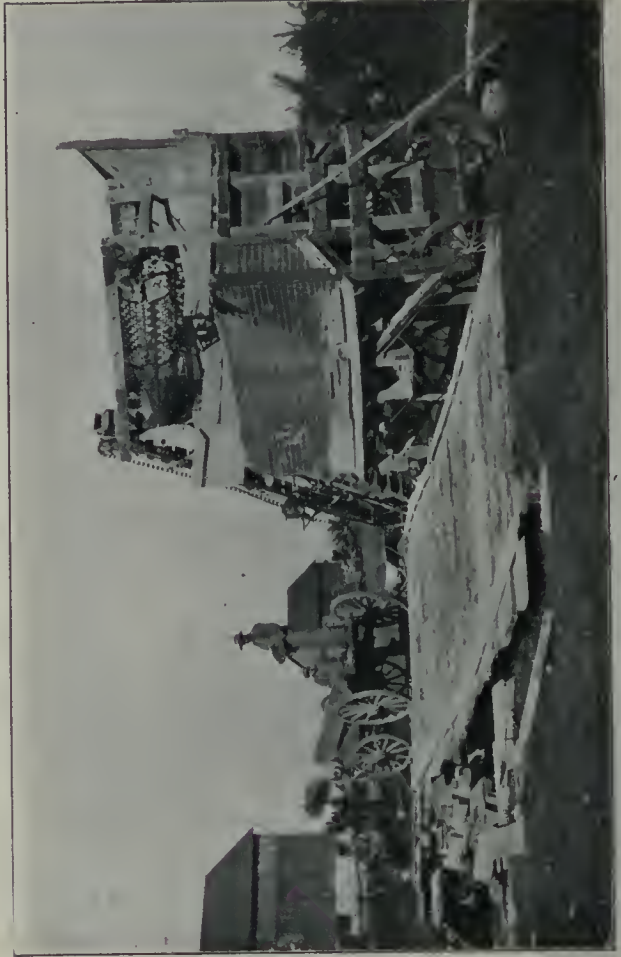
Arrangement of Crushing Equipment—Power from a Traction Engine on top of the bank of gravel; gravel being fed to the Crusher by bucket elevator; material passing through a revolving screen to storage bin.
